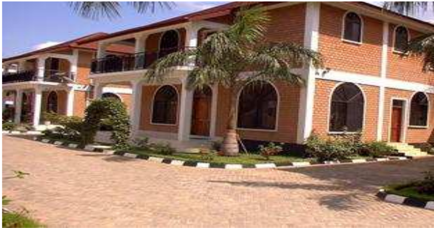
Figure 8. Building with Hydra form Dry Stacked Interlocking Blocks
