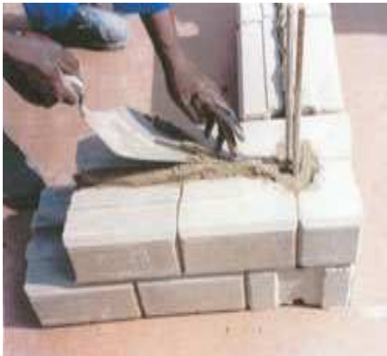
Figure 9. Vertical Steel in Masonry
