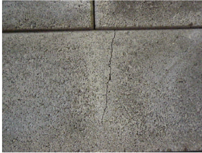
Figure 4—Hairline Crack in CMU
